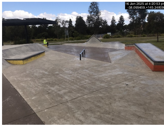
Fig.2 Layout of skatepark, identifying unusual layout and tall hubba on the right.
