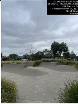
Fig.1 – south to north view
